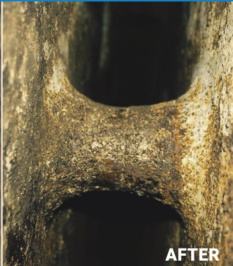
Internal inspection of a cast iron boiler before and after descaling.
