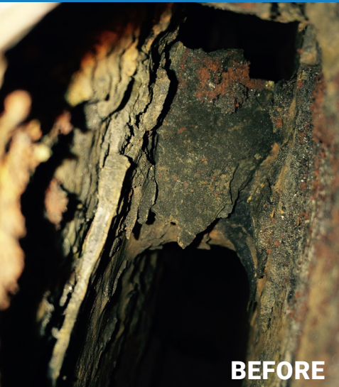
Internal inspection of a cast iron boiler before and after descaling.
